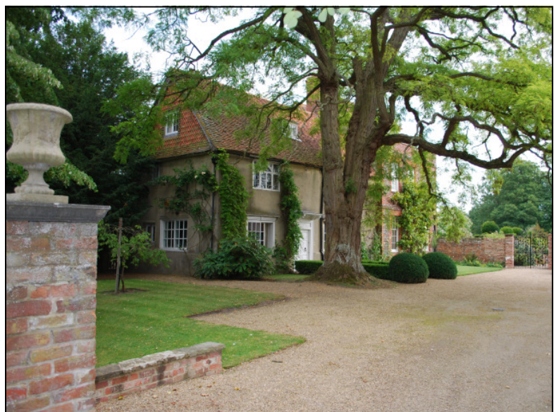
Driveway of Parsonage Farm—2011
